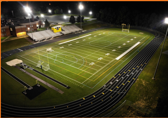
Perryville High School (40) 1500W Metal Halide Flood Lights 14FC Average Uniformity 0.32
